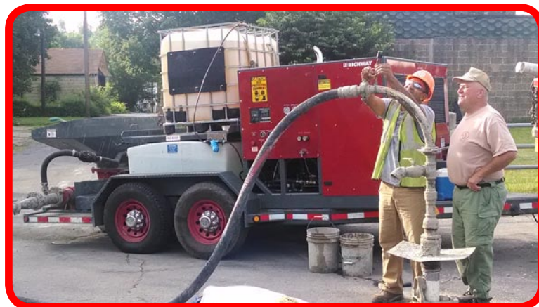
Shown here is a customer with their CT-100D. Cellular concrete is being used for mine abatement within a city to prevent additional subsidence.
