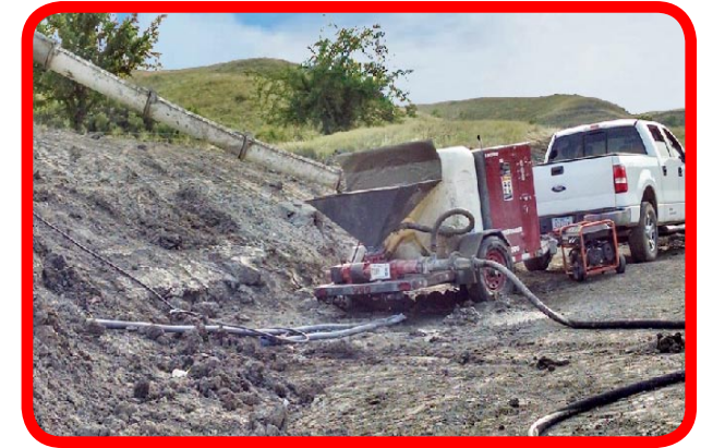
Richway's CT-30G on the jobsite of an annular space fill for a slip lining project.
