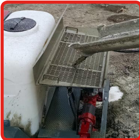
Base slurry being discharged from the ready mix truck into the hopper on a CT-30G
